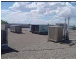
The rooftop units were replaced with more effective equipment.
