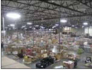
Yearout upgraded the lighting to brighter, more efficient T-5 lights.
